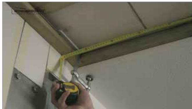
To install the sandwich panels, impregnated wooden battens, a metal stud wall or plastic battens are used. The space between the battens is 1200mm. Use battens with a spacing of 600mm if the ceiling can be touched.
