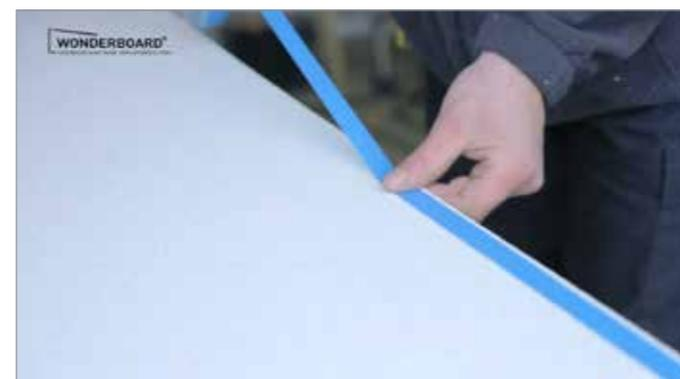
Apply the tape (item no.: 1046) in such a manner that it creates an overlap of approximately 2mm on both sides. This will determine where the 2-component glue will be applied.
