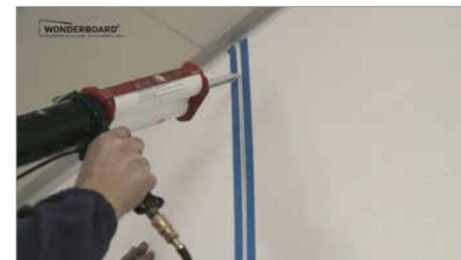
Apply the 2-component glue in the joint from the top to the bottom and check it immediately.
