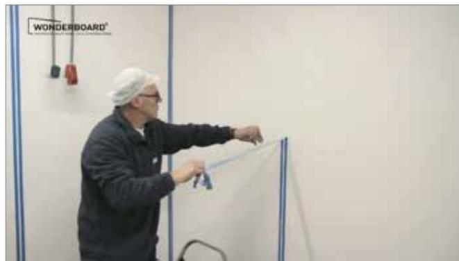
After five minutes, remove the tape from the Wonderboard panel from the top to the bottom.
