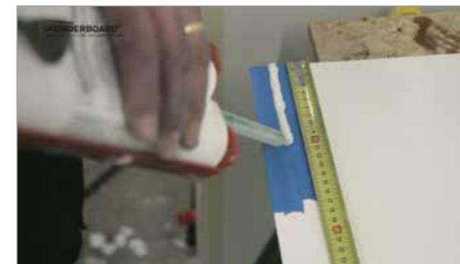
Install the tandem cartridge in the glue gun and dispose of the first 10 cm to ensure the best possible mix is used. Do this with all new cartridges. You should also always use a new nozzle when installing a new cartridge.
