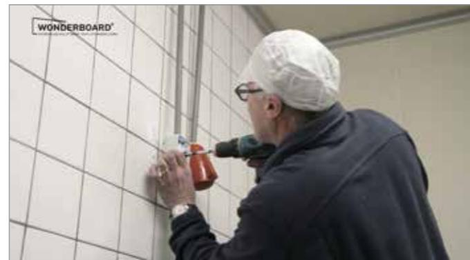
It is recommended to remove all obstacles before cleaning the walls. This will allow for quick and effective cleaning and installation. Depending on the size of the obstacles, they can later be finished using the required profiles, sealant or 2-component glue.
