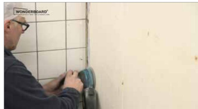
The current sandwich panels often have rust spots. Sand these rust spots. Remove any loose paint and coating layers using a putty knife and sand these spots as well using a sanding machine. Then lightly sand the remaining part of the wall.
